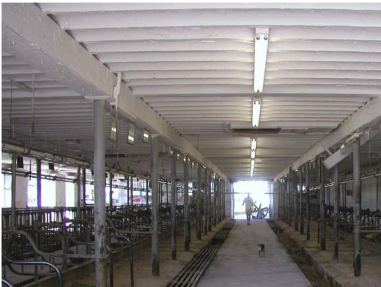
Figure 2. Interior Photo of Two Story Dairy barn with two rows of posts and beams.
